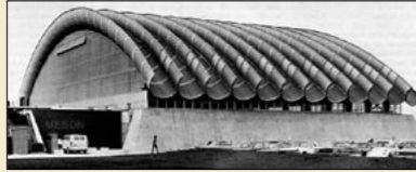
The Meson hall houses the bulk of the detection systems for experiments on secondary beams with energies up to 300 GeV. The beams, emerging from a single target, enter from the left and "fingers" to accommodate additional detectors protrude behind the building on the right.
